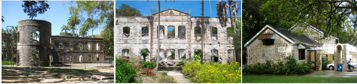
Figure 96. Farley Hill Park Great House (left and middle); associated buildings (right).
