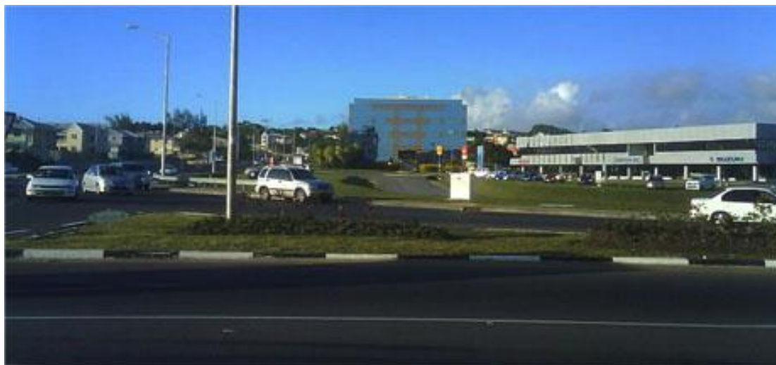
Figure G6. The upgraded intersection at Darcy Scott Roundabout linking the ABC and Ronald Mapp Highways.
