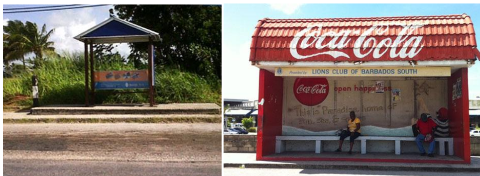
Figure G3. Bus shelters outside of the GAIA compound. Sponsors should be asked to rebuild these shelters to conform to current airport design.
